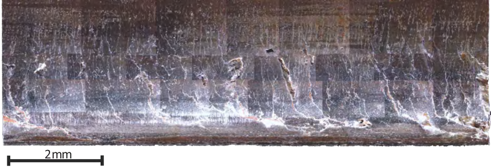
Figure 2.5: Head checks on the gauge corner of the rail.
