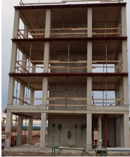
Figure 2. Overview of the large concrete structure SKUSTA without test objects; during testing all compartments were filled with various test objects (photo used with courtesy of the SHIELD group)
