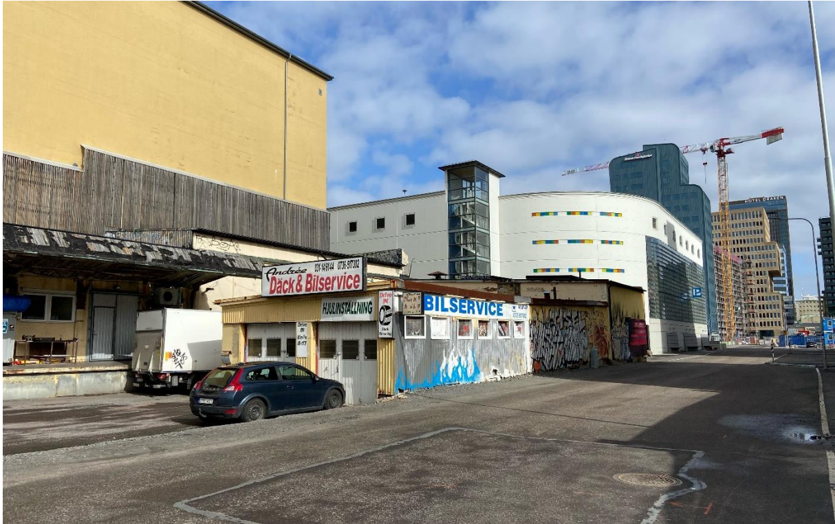
Figure 3: Masthamngatan—which runs right through the redevelopment area—is slated to become a pedestrian-friendly street with active frontages and diverse outdoors amenities. Ongoing construction visible in the background. Image: Author’s own.
