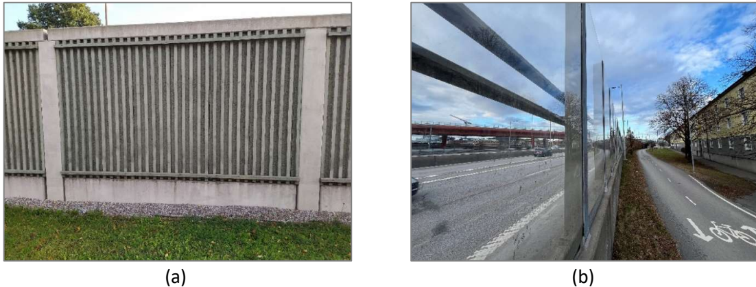
Figure 3 3: (a) Concrete noise barrier with sections of inlayed absorbers, (b) transparent noise barrier.
