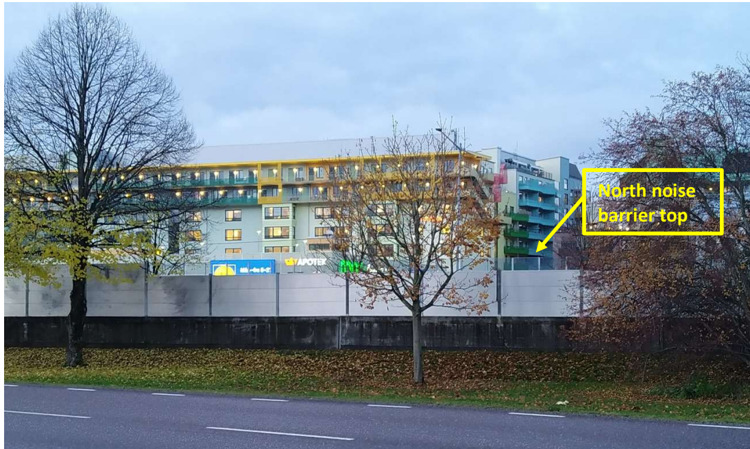
Figure 4.3: The second site, behind a 3.0-3.6 m tall noise barrier south of the motorway. Above the barrier, some of the new buildings and the top of the new 5.4 m tall noise barrier north of the motorway can be seen.
