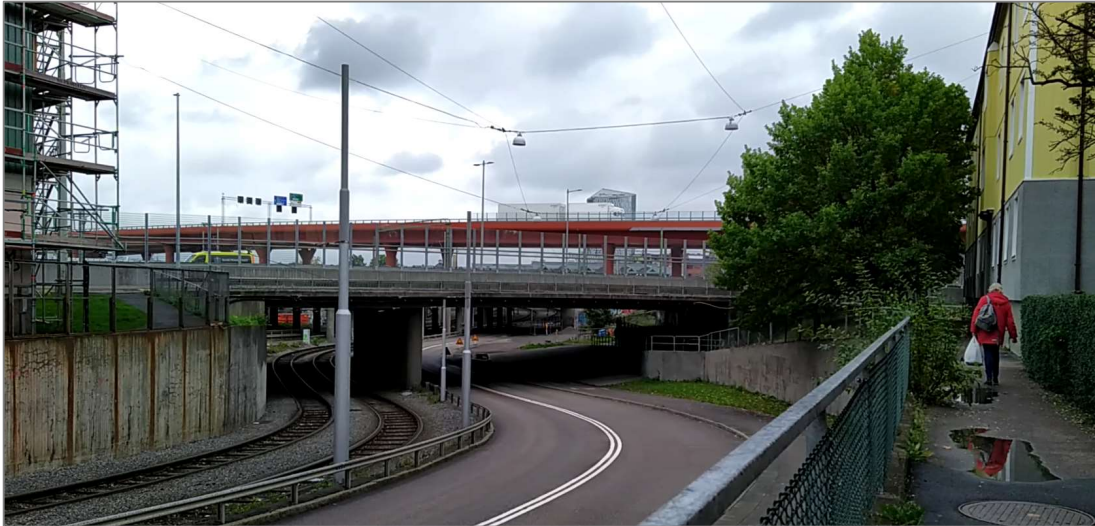
Figure 1.2: Several levels and dimensions of traffic infrastructure in a Swedish urban area.
