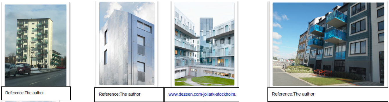
Figure 18. The figure depicts a collection of buildings featuring façades that interact with sunlight through mirror or reflectance effects. The interplay of the sun with the façade produces a striking effect and lightens the chosen color’s hue on the façade where direct sunlight is present.
