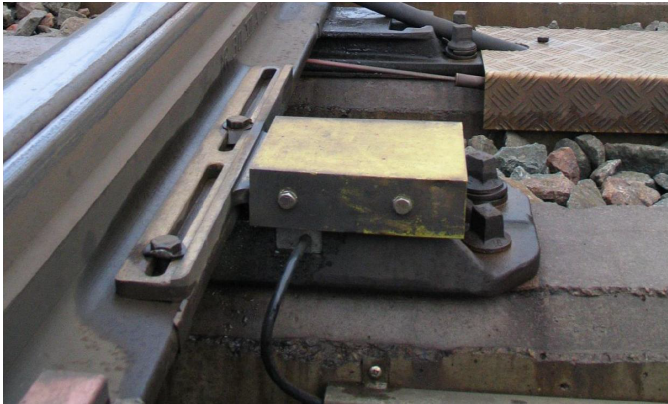
Figure 1.3: TKK sensor in track [11]
