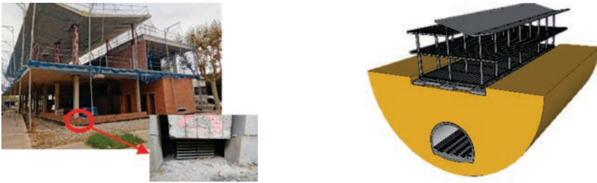
Figure 50-1 General overview of the vibration isolation case study: left: physical building; right: numerical model.
