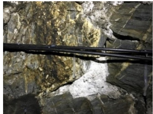
Figure 55-2 Fixation with facing irregularity
