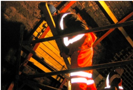
Figure 74-1 Traditional method of undertaking tunnel brickwork repairs
