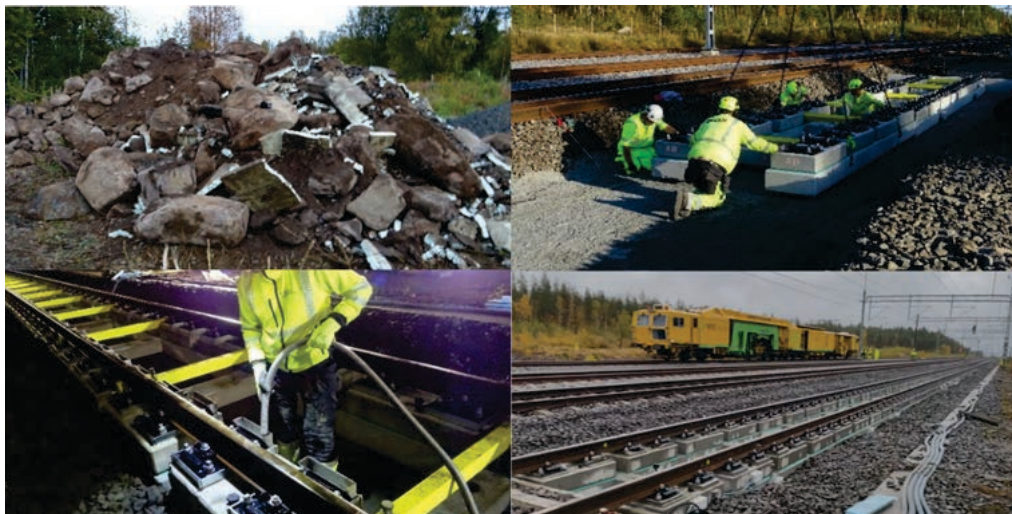
Figure 62-3 Large boulders found during excavation (upper left), whole modules being positioned (upper right), pouring of levelling mortar (bottom left), finished track section at 96 hours (bottom right).
