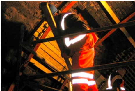
Figure 74-1 Traditional method of undertaking tunnel brickwork repairs
