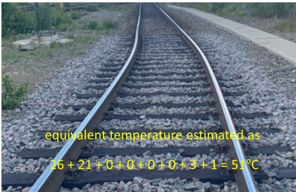
Figure 24-1 Track buckle with corresponding evaluation of equivalent temperature as a sum of contributing factors. Picture Trafikverket.
