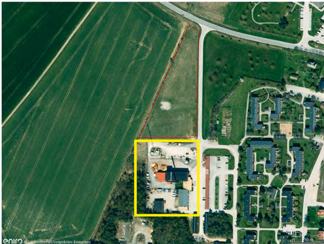
Fig. 2. Boiler central – Satellite photo of the Hemse boiler plant (yellow square) and surrounding area. Available land for installation of solar collectors are located to the north. (For interpretation of the references to colour in this figure legend, the reader is referred to the web version of this article.)
