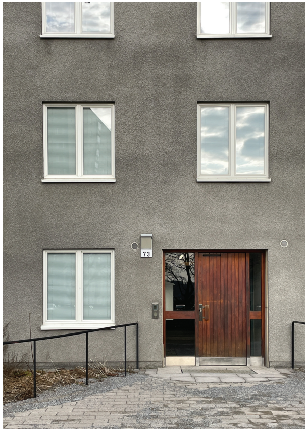
Figure 4. Windows of Valla Gärde in alignment with the façade after renovation.
