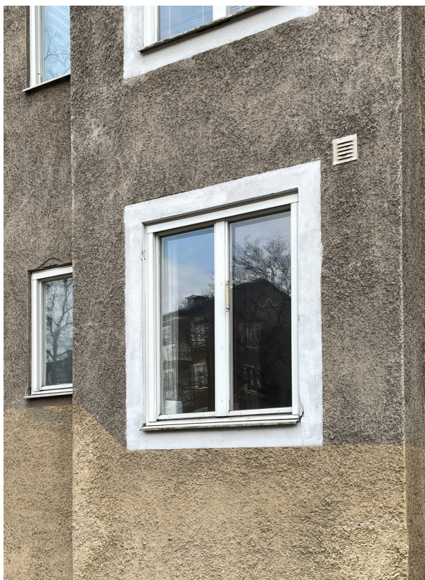
Figure 5. Window arrangement before external thermal insulation in Solberga.
