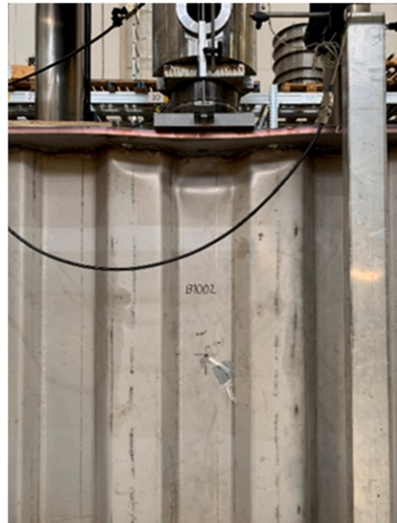
(b) Girder SSCWW300
