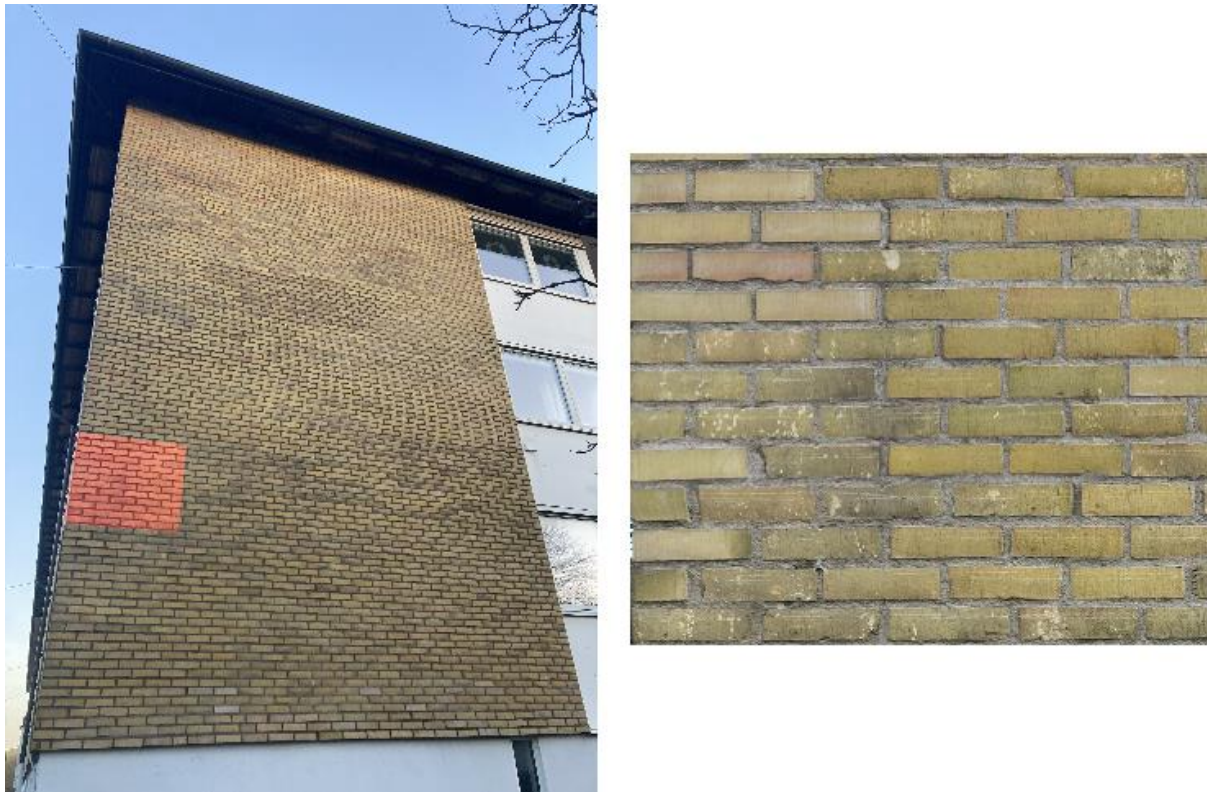
Figure 18 Photograph of Facade 2 (the validation facade). On the right is a detailed view of the area marked with a red mask in the photograph, illustrating replaced bricks and bricks undergoing spalling.
