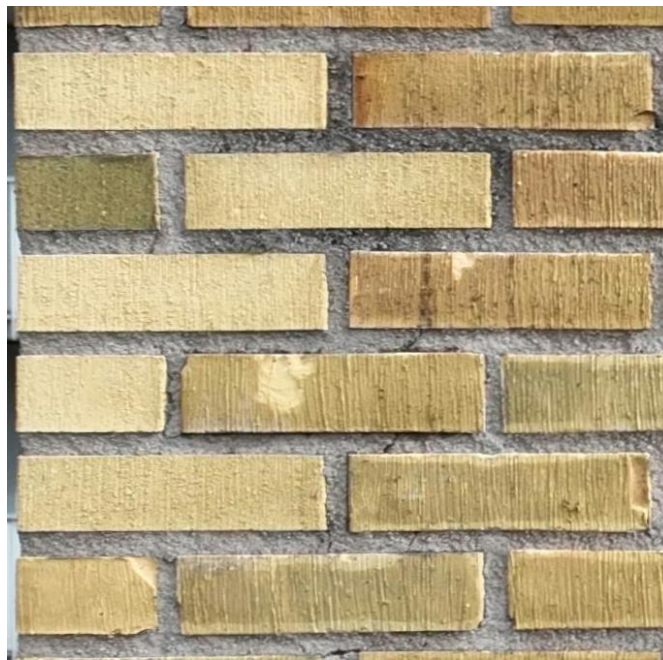
Figure 7 Example of the spalled and replaced bricks (bricks of noticeably brighter color) on a facade from the case study. Both are considered degraded for further analysis.
