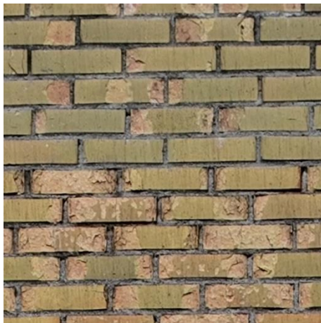
Figure 3 The effects of microclimate. Photograph on the top shows the brick part of a facade in Flatås, Gothenburg, Sweden. On the bottom left, there is a detailed view of the facade, showing bricks subjected to spalling. The drawing on the bottom right shows the facade situation with respect to the surrounding buildings.
