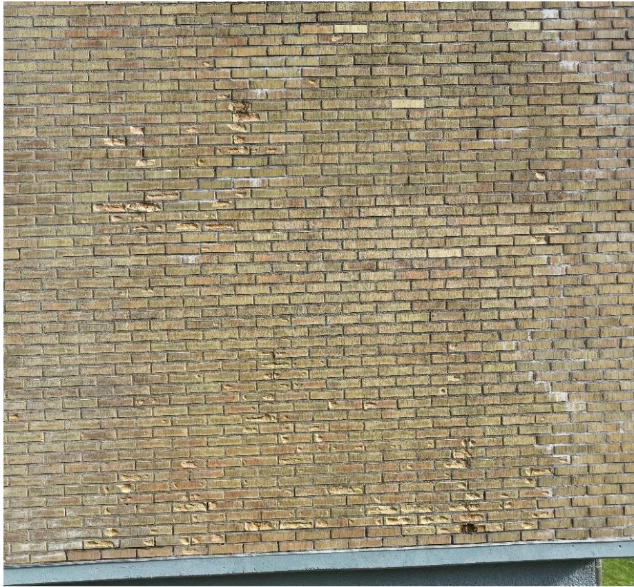
Figure 2 Localized spalling degradation on a brick facade of a residential building in Gothenburg, Sweden. The facade was renovated in 2013.
