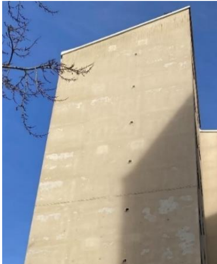
Figure 1 Localized delamination of render on a high-rise building in Gothenburg, Sweden. The degradation occurred approximately 10 years after a major renovation of the building's facade.
