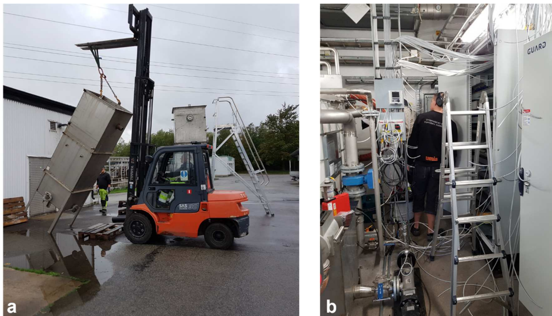
Figure 3. a) Mounting of the reactors for hydrolysis and fermentation. b) The pilot plant room during electrical installation.
