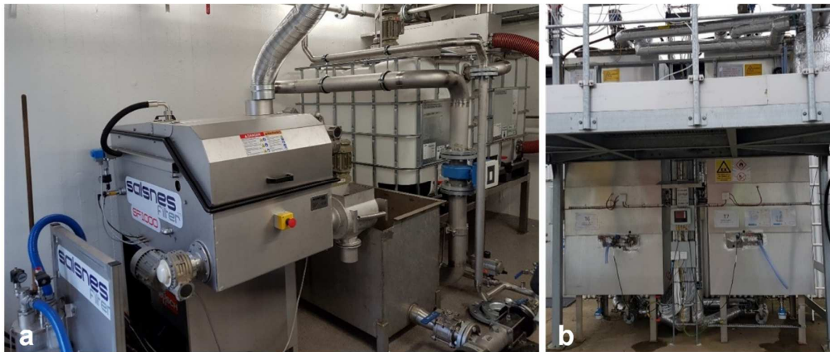
Figure 4. a) Flocculation tanks and rotating belt filter at the ICU pilot plant for wastewater primary treatment. b) Fermentation reactors.
