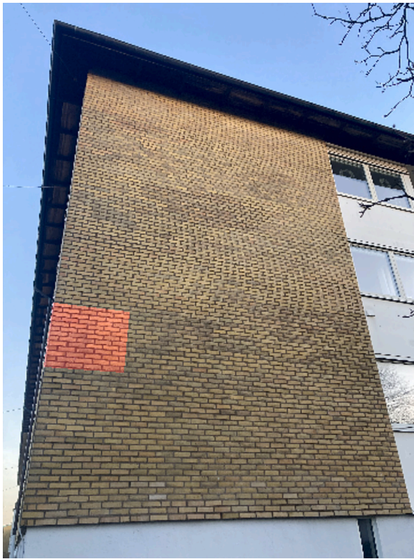
Fig. 11. Photograph of Façade 2 that is hereafter regarded as the validation façade for testing the ability of the predictor to generalize to unseen data, which may be drawn from different degradation distribution. Right: detailed view of the area highlighted with a red mask in the photograph, showing bricks undergoing spalling (lighter-colored areas inside bricks). Bricks with a lighter overall appearance, mostly located on the left side, are considered as replaced bricks in further analysis. (For interpretation of the references to colour in this figure legend, the reader is referred to the web version of this article.)
