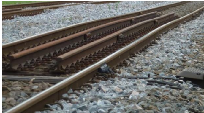
Figure 3.1. Transition zone with auxiliary rails and a large differential settlement, from [5].
