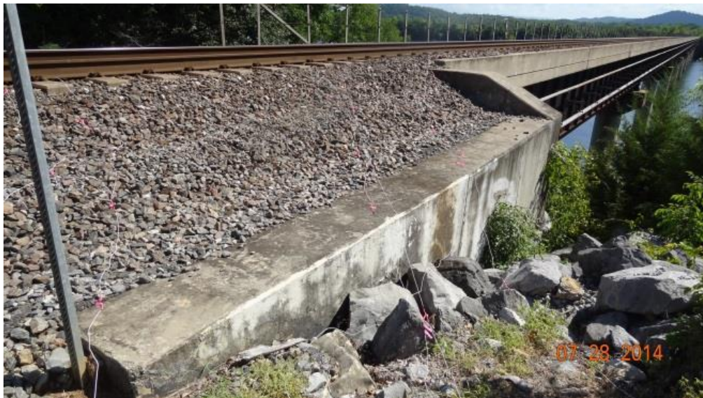
Figure 3.11. Bridge transition zone with concrete confinement wings walls parallel to the track. From [78].
