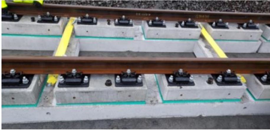
Figure 4.2. A view of the 3MB slab design consisting of base slabs, top blocks, and an elastomeric layer between the concrete layers.
