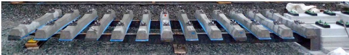
Figure 3.12. The universal transition module V-TRAS pictured as it is provided, supported on the massive end of the ballastless track and floating on the ballast bed [79].
