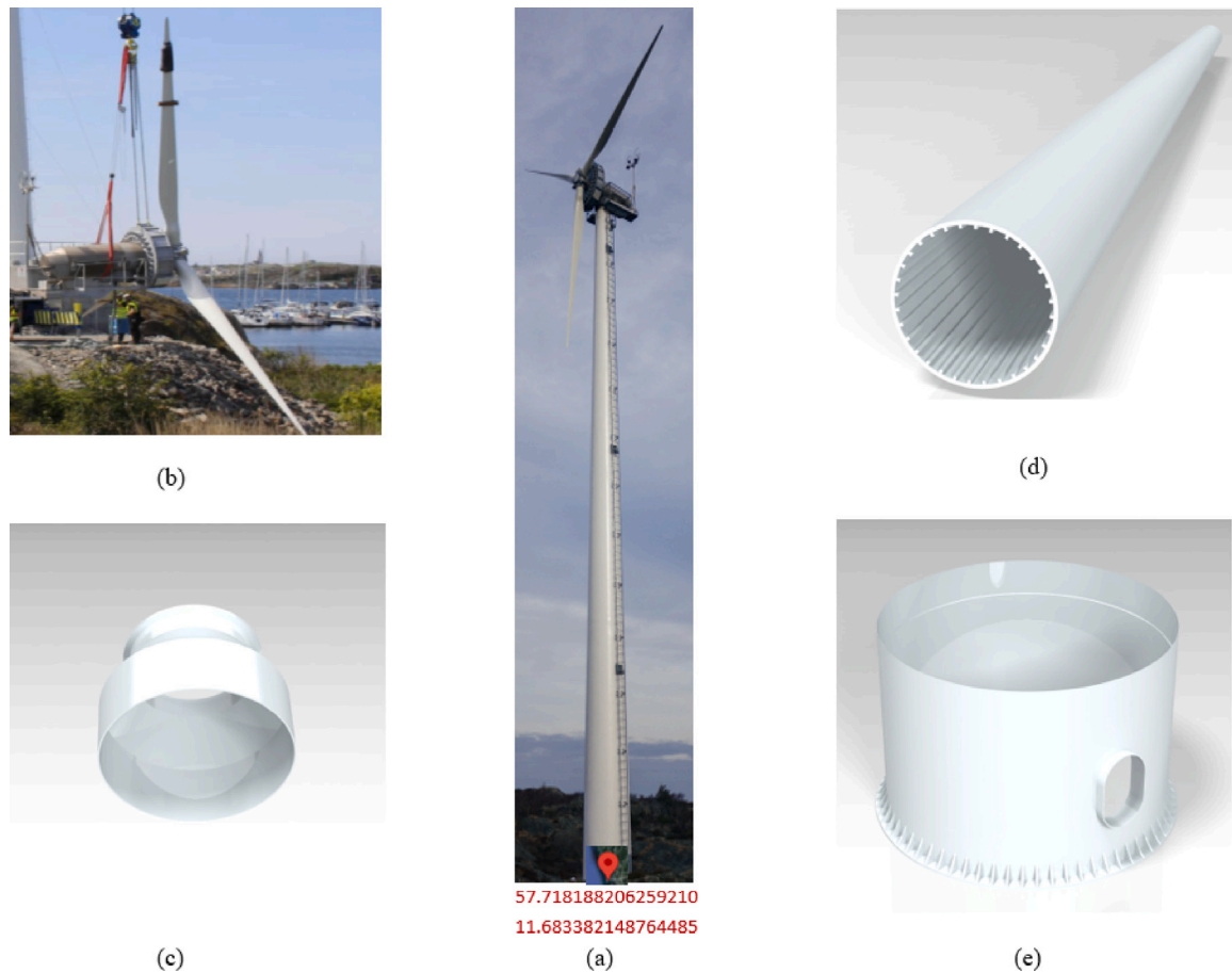
Fig. 1. Chalmers wind turbine and its components: (a) Geographic coordinate, (b) Rotor Nacelle Assembly (RNA), (c) Steel top adapter, (d) CAD model of wooden tower body, (e) CAD model of Steel base.
