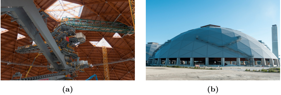
Figure 2.10: Reticular dome in Brindisi, Italy. (a) internal view, (b) external view. Rubner. Photo: Oliver Jaist Fotografie
