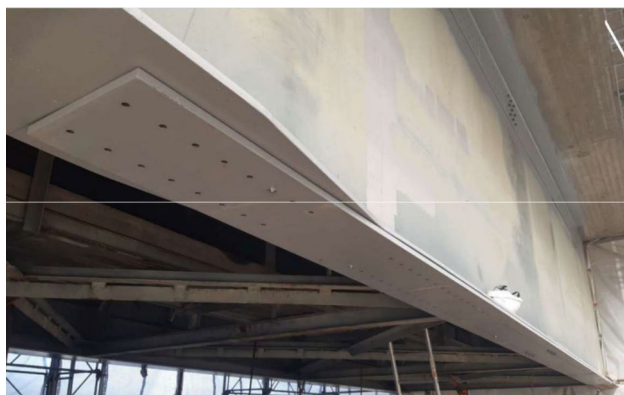
Fig. 1 An example of a beam cover plate that has been prepared for bolting onto an existing bridge girder
