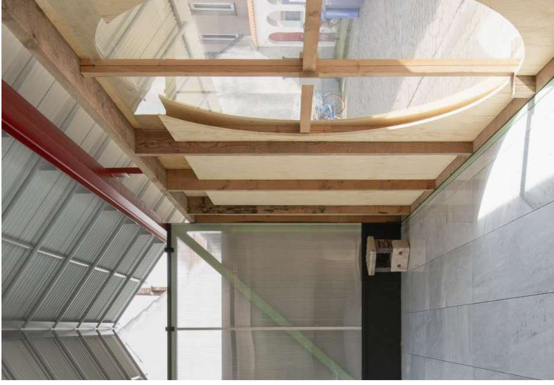
Norell/Rodhe, Raamland (2024). The design and construction were based on reclaimed materials gathered from various contexts, including wall panels from an abandoned club in Oostende, second-hand Carrara marble tiles from Brussels and timber studs and plywood sheets from previous triennials.
