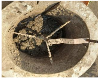
(b) Inlet status indicating inconsistent feeding and cleaning.
