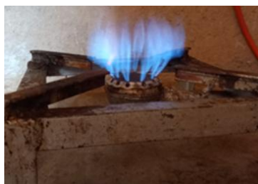
(c) Stable blue flame, indicating less impurities and good combustion from quality biogas.
