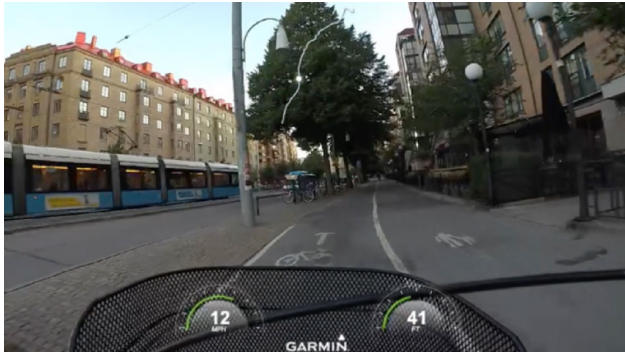
Fig. 14 Cycling path in Gothenburg with patches and bad pavement
