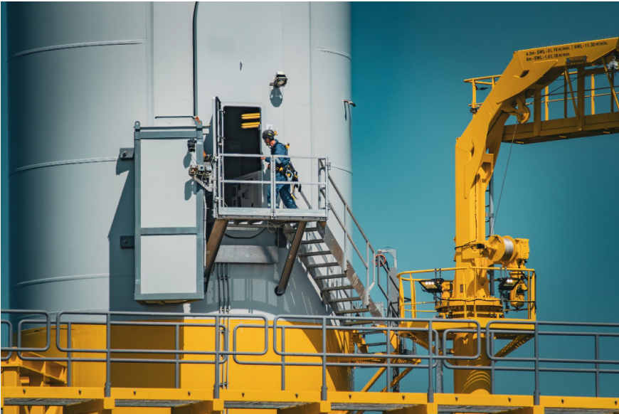
Fig. 16: A worker accesses the base of the tower on one of the Kincardine FOWTs (Photo Credit: Flotation Energy)
