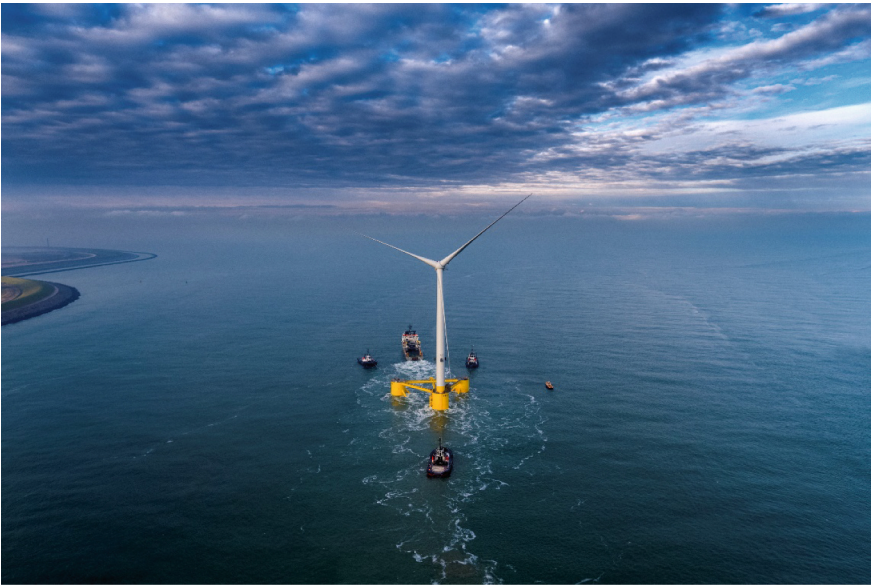
Fig. 15: One of the Kincardine floating wind turbines being towed to site illustrating the multiple vessels required for a relatively small FOWT (Photo Credit: Flotation Energy)
