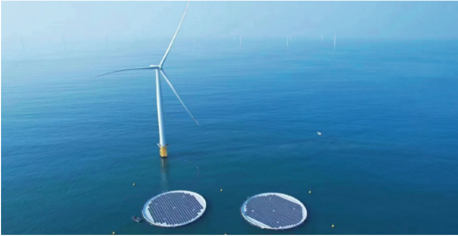
Fig. 36. Hybrid offshore wind-solar power plant. Adapted from (Garrod et al., 2024).
