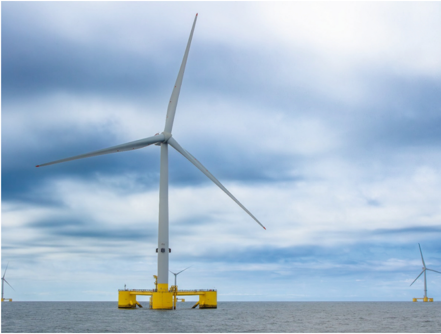
Fig. 7: Kincardine offshore wind farm, showing three of the five 9.5 MW Vestas wind turbines on steel semi-submersible foundations designed by Principle Power (Photo Credit: Flotation Energy)
