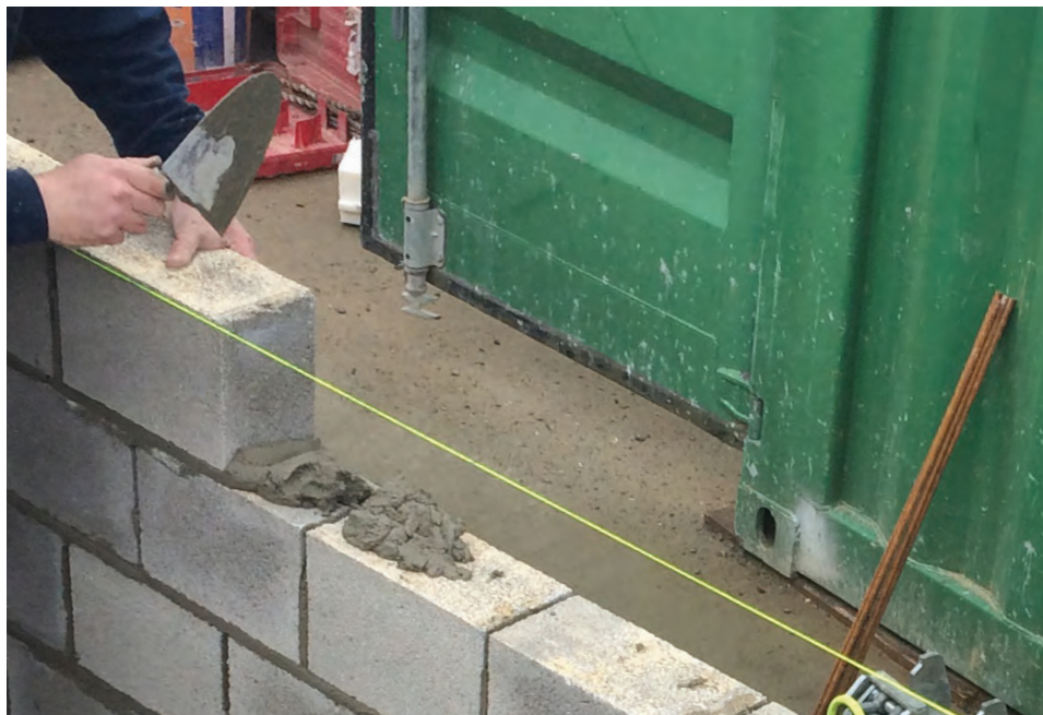
The actions of wall-making following the guiding lines
