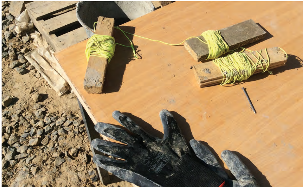
ill. 4.13: Wrapped lines ready for action and waiting to put Euclid's constructive principle at work: traced, extended, attached and tensioned to enact a line from nail/ point to nail/point
