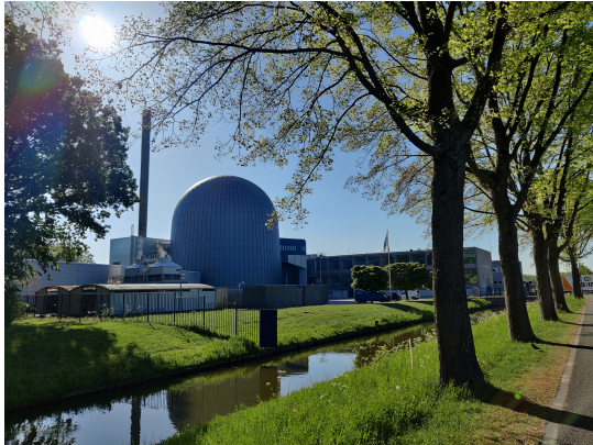
(a) TU Delft, the Netherlands
