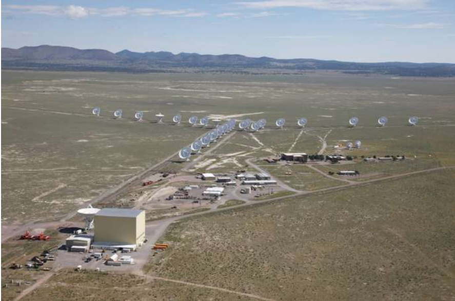
Figure 1.4: The Karl G. Jansky Very Large Array (VLA) located on the Plains of San Agustin in New Mexico, USA. The array consists of 27 antennas arranged in a Y-shaped configuration, providing baselines up to 36 km and enabling high-resolution radio imaging. Image credit: NRAO/AUI/NSF.
