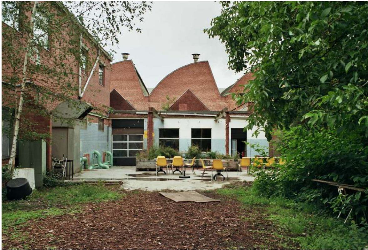
Fig. 56: The back of the Blikfabriek site, located next to the Blikvelden wetland.
