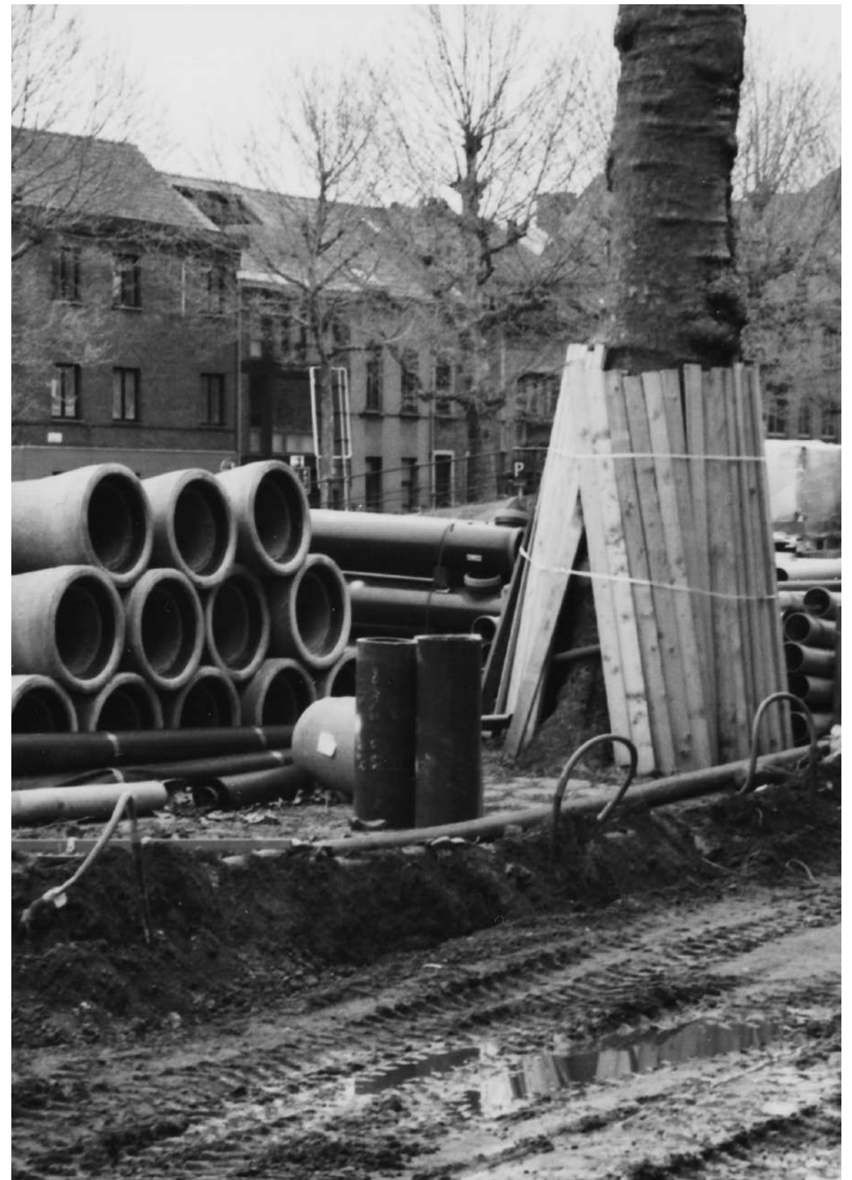
Fig. 5: Image of large-scale sewer construction in Ghent, Belgium, with the pavement being removed from the soil and sewage pipes awaiting implementation, while trees are protected from the construction works.
