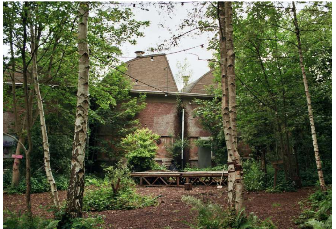
Fig. 59: The back of the Blikfabriek site, located next to the Blikvelden wetland.
