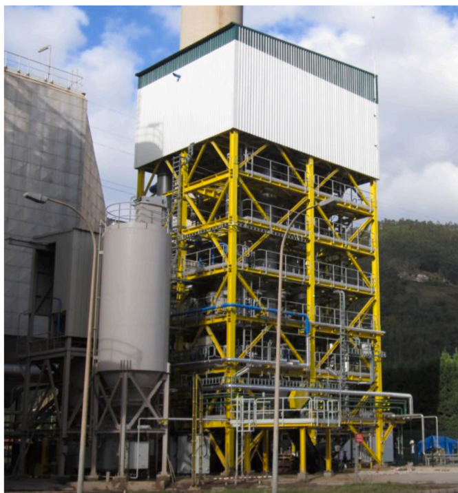
Fig. 11. Photograph of the 1.7-MW th La Pereda pilot plant connected to an existing 50 MW e power plant. Adapted from Diego et al. (2016a) with permission.
