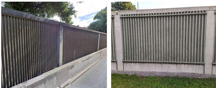
Figure 3.20: The noise barrier at Site 3. To the left, corrugated concrete surface on the roadside (photo: Akustikkonsulten), to the right, wooden slats with cement-bound wood wool panels (photo: author).
