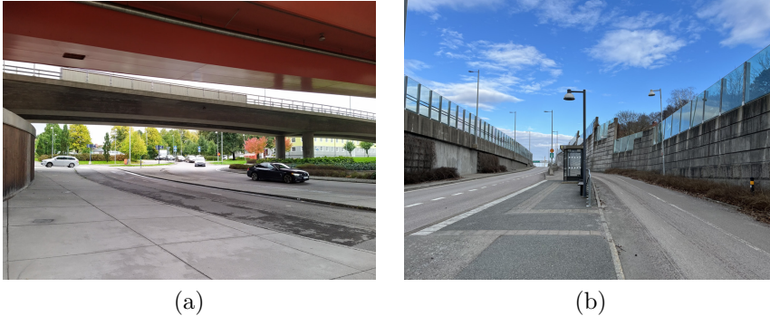
Figure 2.1: (a) Concrete and steel motorway bridges over a local street, (b) urban road canyon (motorway ramp, bus stop and bike lane), with supporting walls and noise barriers.
