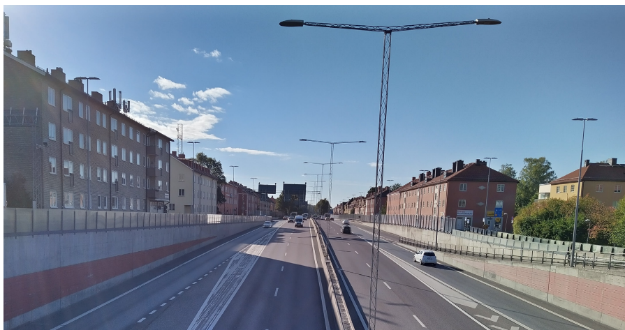
Figure 3.19: View over the 6-lane road at Site 3, flanked by noise barriers and apartment buildings. The receiver positions for the measurements and calculations are situated further down the road on the left hand side.
