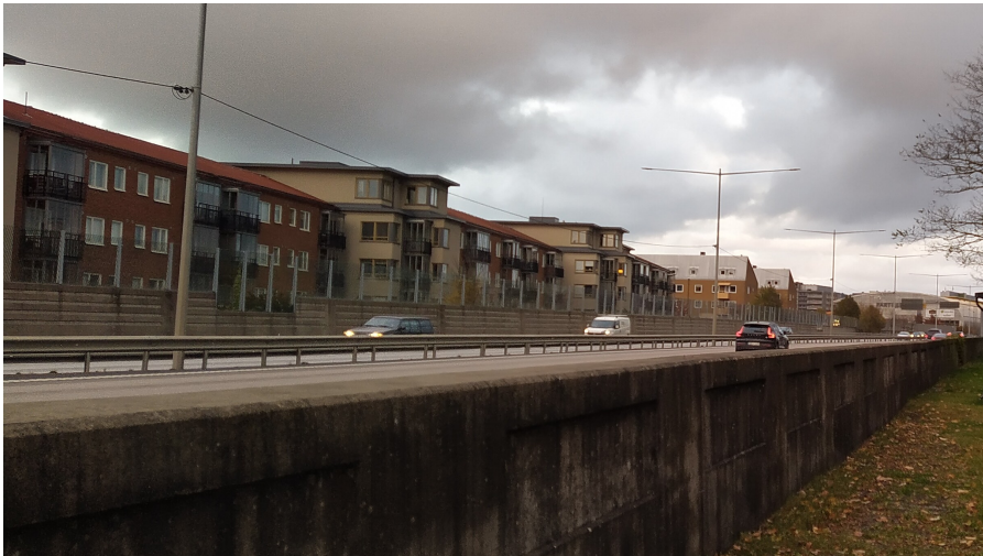
Figure 3.1: Site 1 seen from the opposite side of the six-lane motorway.
