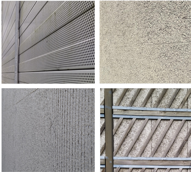
Figure 4.9: The absorber and noise barrier types: perforated metal cassette with mineral wool (top left), porous concrete (top right), LDPE foam panel (bottom left) and cement-bound wood wool sheets (bottom right).
