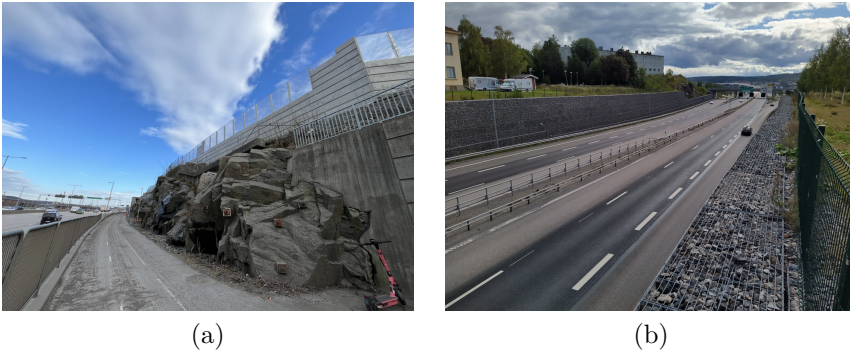
Figure 2.2: (a) Concrete and polycarbonate noise barriers on top of rock cutting, (b) claddings of stone gabions on rock cuttings and supporting walls.
