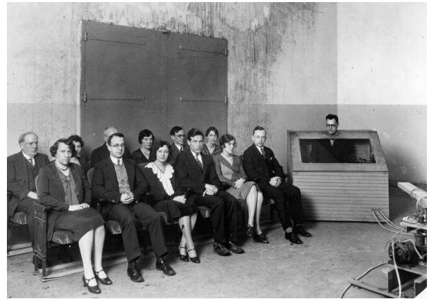
Figure 4. Measurement of the influence of the presence of people on the reverberation time [4].
