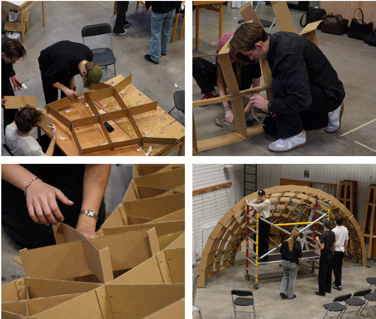
Figure 7: Incremental assembly of the first arch segment. Top left: assembly of an individual zone. Top right: joining of two zones in the arch. Bottom left: installation of bracing members in the end bay. Bottom right: completed arch segment ready for connection to subsequent arch segments.
