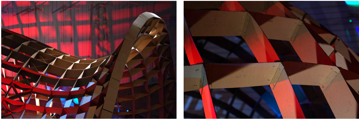
Figure 9: Details of the completed cardboard gridshell. Left: surface geometry across a region of the pavilion. Right: close-up of a node connection showing the integrated folded end-crease detail.
